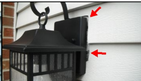
Caulking to prevent moisture/pest intrusion.
