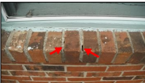
Mortar joints deteriorating
