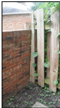
Outside fence board cut at an angle to accommodate leaning retaining wall
