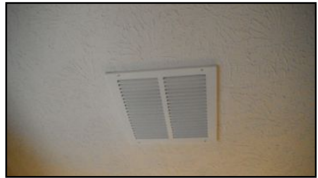
Upstairs bathroom exhaust vent
