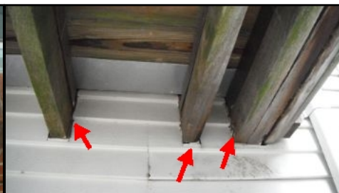
Caulking to prevent moisture/pest intrusion
