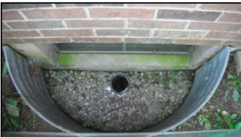
Basement Window Well, drain noted
