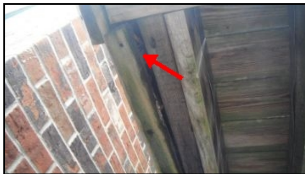
Cantilever balcony floor joist is rotting
