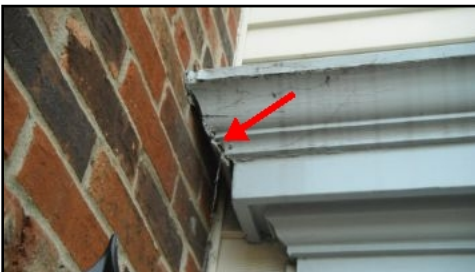
Caulking to prevent moisture intrusion
