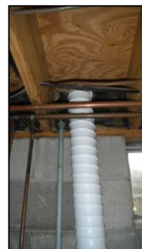
Dryer flex hose going out through box sill
