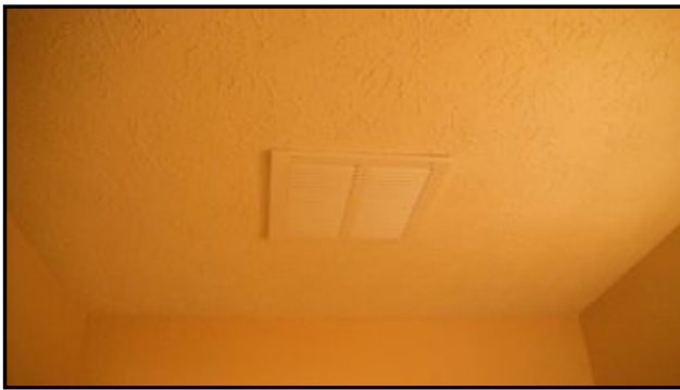
Upstairs bathroom exhaust vent
