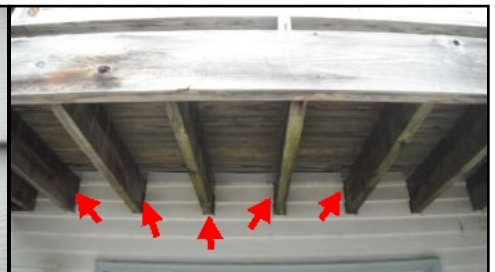
Caulking to prevent moisture/pest intrusion
