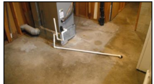
Condensate line from furnace going in to floor drain
