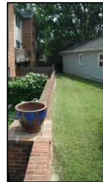
Retaining wall is leaning inwards
