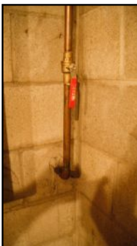
Water shutoff valve in utility area in basement
