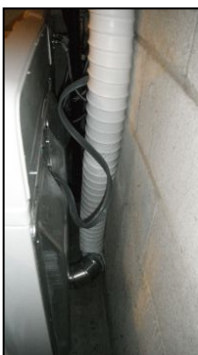
Dryer flex hose coming out of dryer
