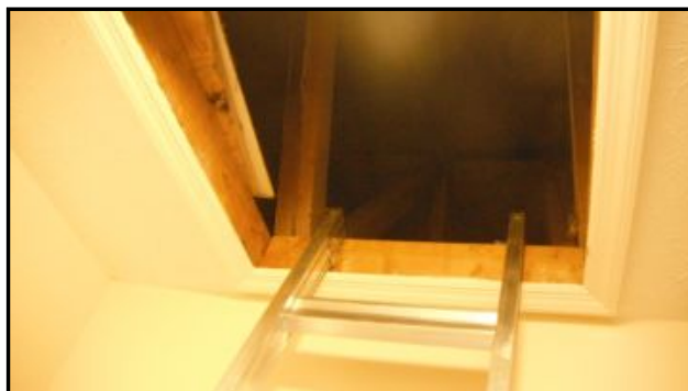
Suggest adding insulation to back side of access panel
