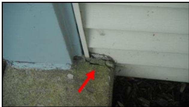
Concrete chipping/cracking
