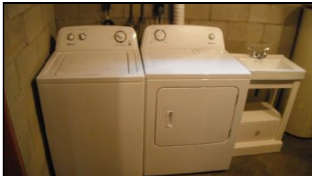
Wash Basin is not connected to plumbing
